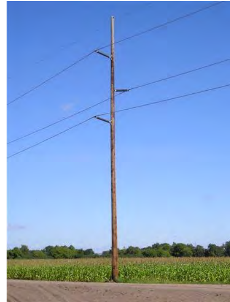
Typical 115-kV wood single circuit structure
