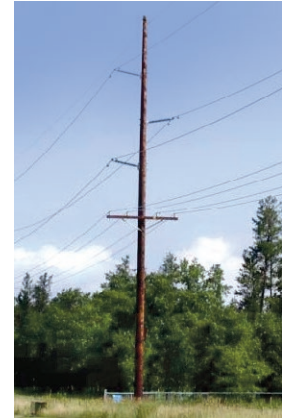
Typical 115-kV wood single circuit structure with and without distribution under build.
