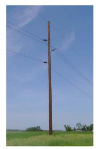
Typical 69-kV single circuit structure
